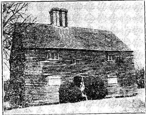
It looks old and it is old. House at Cutchogue is believed to have been built more than 300 years ago.
