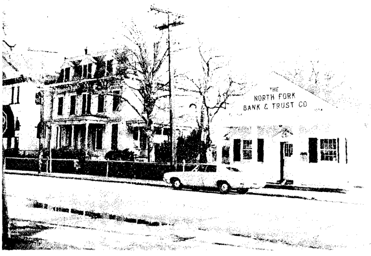
ITS DAYS ARE NUMBERED: the graceful and sturdy Klipp house stands next to the present Greenport branch of the North Fork Bank and Trust Company on Main Street. The bank is planning to raze the nearly 150-year-old building to replace it with a modern brick and clapboard structure to house the business that has doubled in the last ten years.
